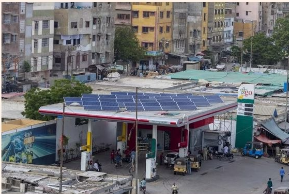
Petrol station with solar plates on its roof in Karachi © (c) Maqibyasir | Dreamstime.com
